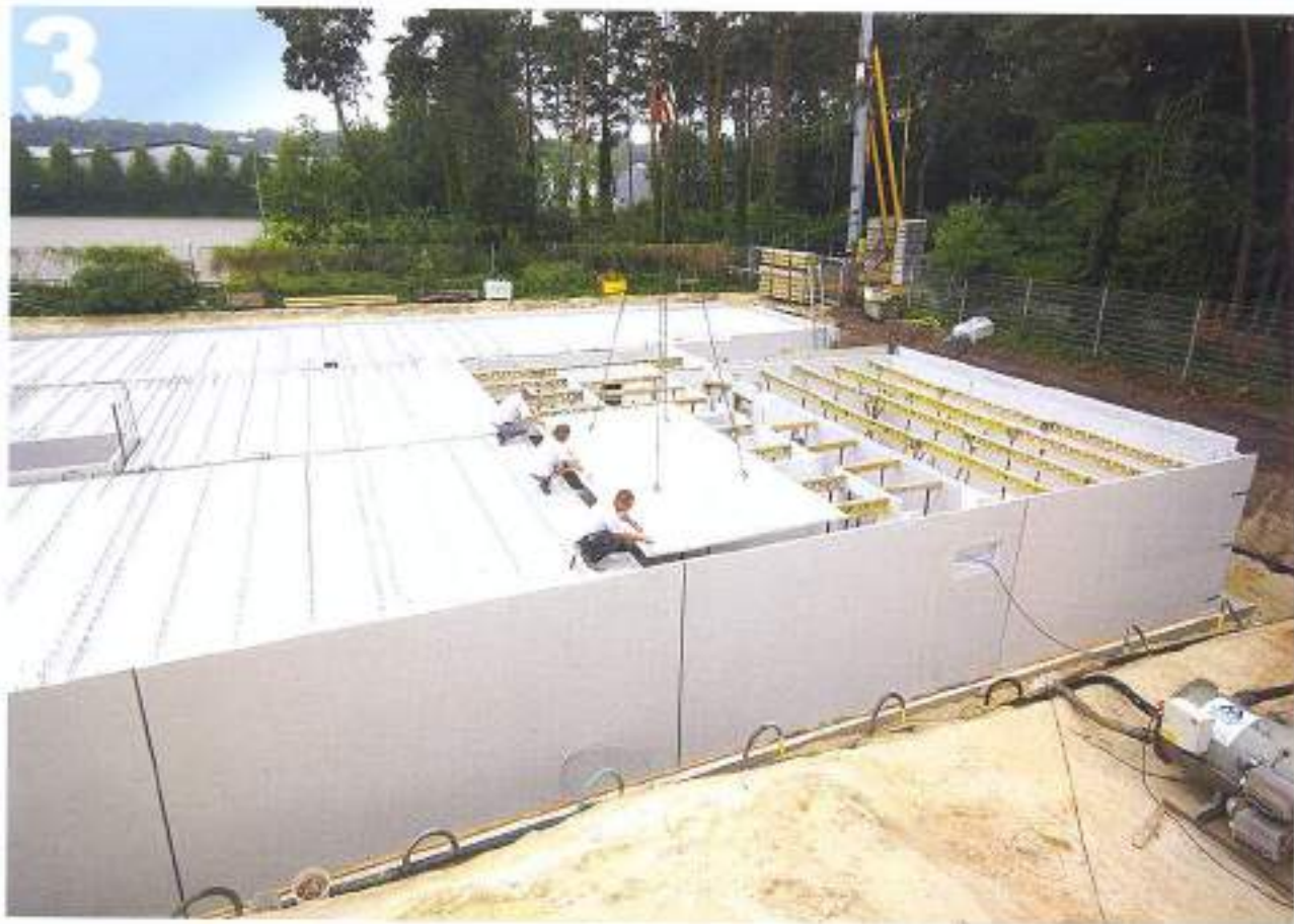
The under side of Emfil Slabs is as smooth as the outside of the " Emfil Walls " seen in this photo. Some Emfil Slabs at the left side are equipped with additional lattice girders to take care for specific structural requirements.
