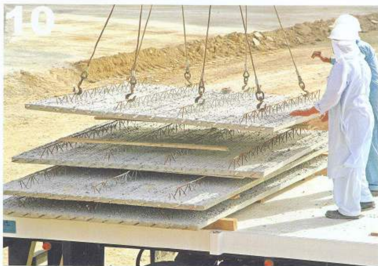
Emfil Slabs are light compared to any other precast concrete floor element. Handling of Emfil Slabs is easy and safe. Gear hooks are connected to the lattice girders.
