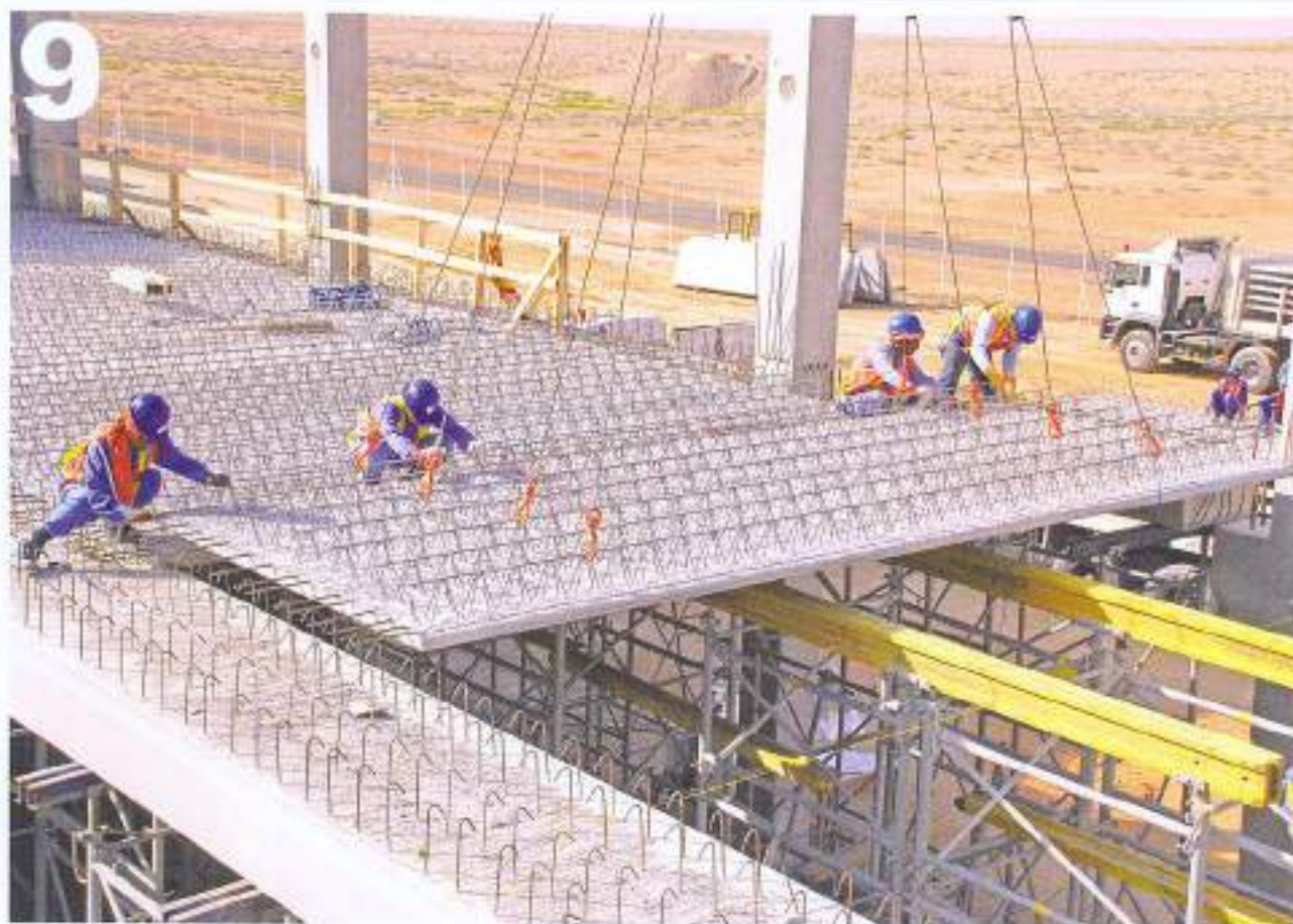
Emfil Slabs speed up the building process. Usual construction steps are reduced to halve. Contractors highlight especially savings in plywood and elimination of moving shattering in and out of each floor.
