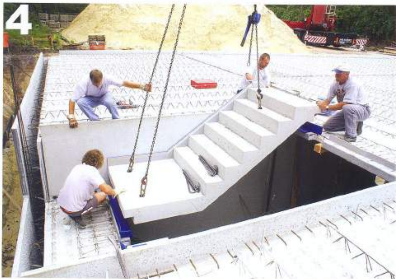
A precast stair element is placed into its final position. Especially of interest is the easy integration of this Emfil Stair element into the structure based on Emfil Slabs . Good to see are Emfil Walls at the left side.
