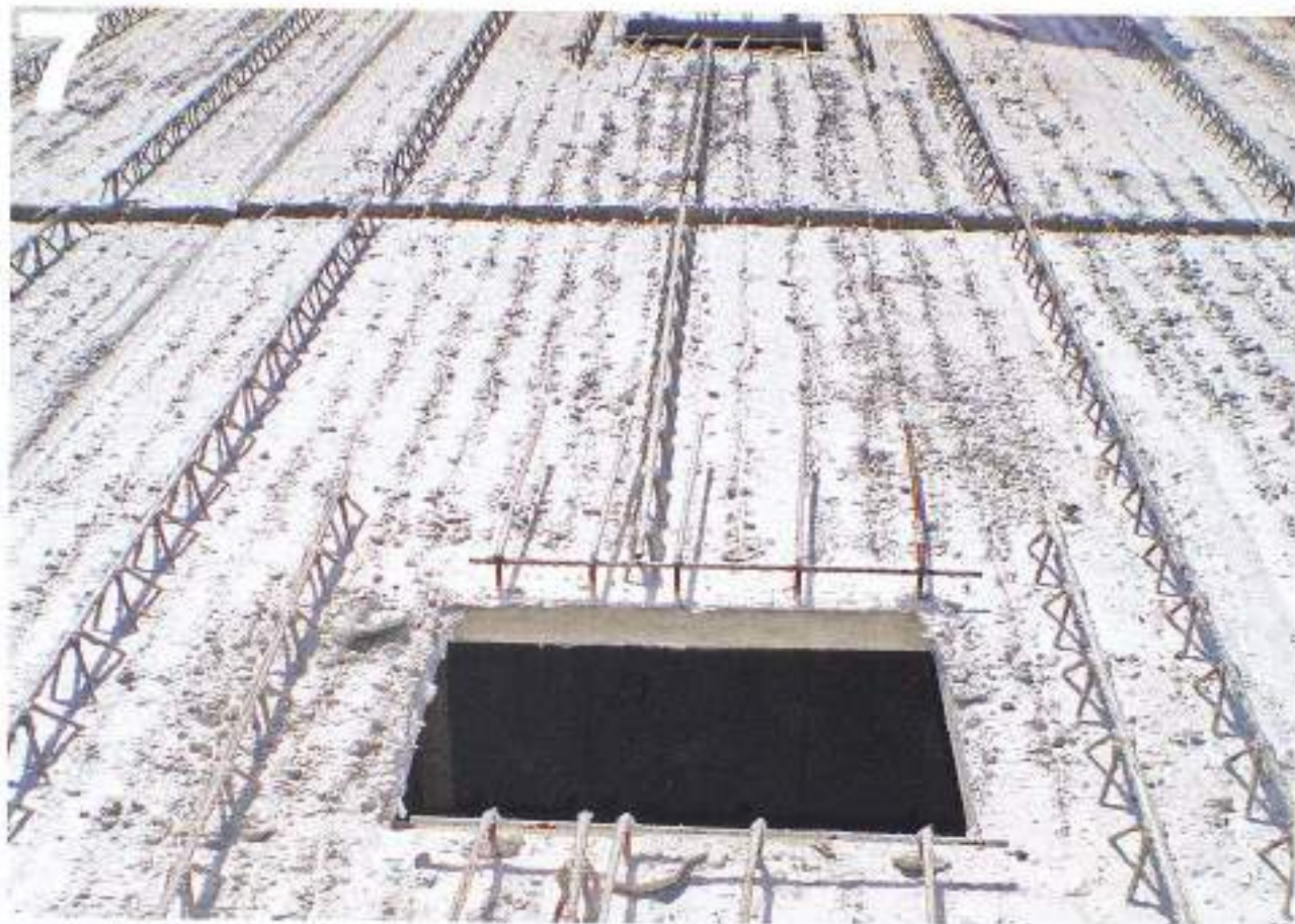
Emfil Slabs offer the designer nearly unrestricted ground plan possibilities. All necessary recesses are made at the correct places in the factory.
