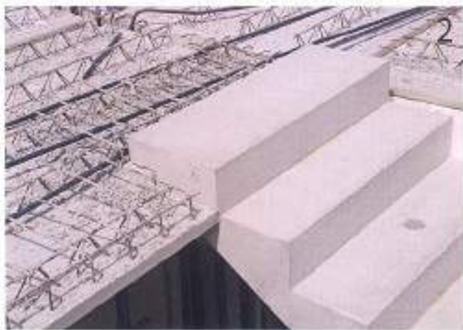
Emfil Stair connected to Emfil Slab
