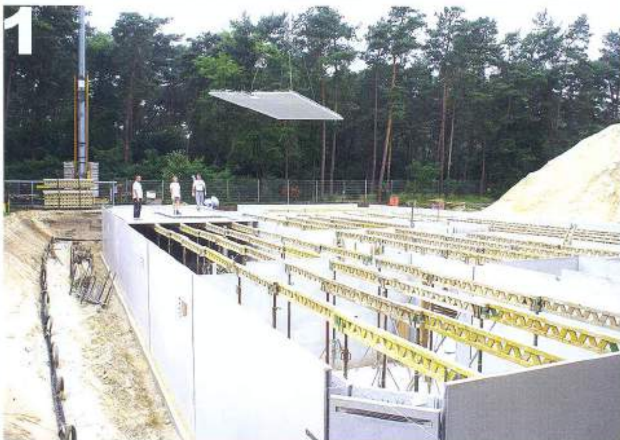
Support girders are placed in position. Some Emfil Slabs are already laid. Basement walls are "Emfil Walls". Emfil Slabs are placed on to the inner shell of the Double Walls, therefore no girder along the walls.
