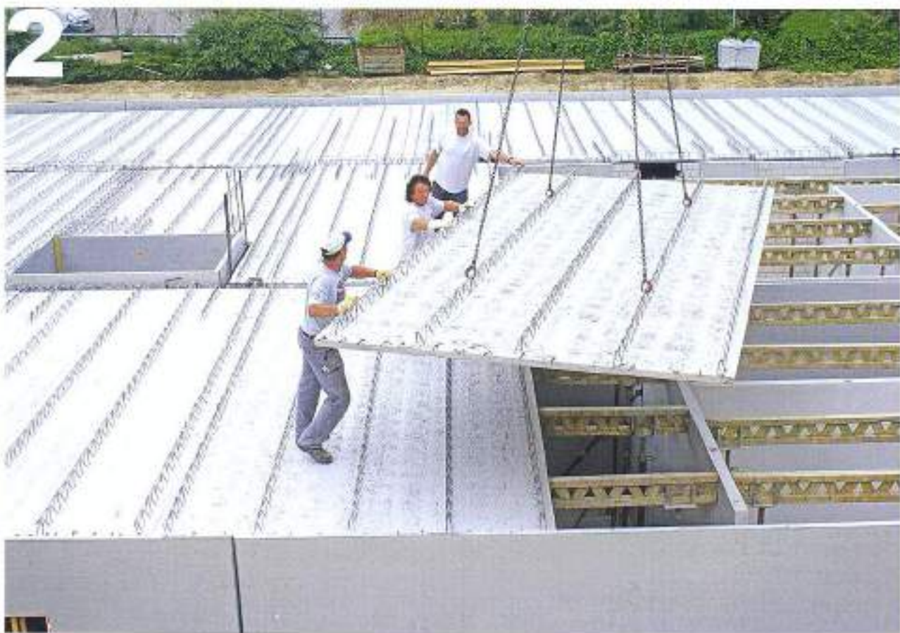
Large Emfil Slabs can be produced and laid due to their low weight per m^2 (in this case the slab is 5cm thick and weighs 125kg/m^2 ). Light cranes can usually handle villa sites. Handling is safe as 4 hooks are connected to the lattice girders.
